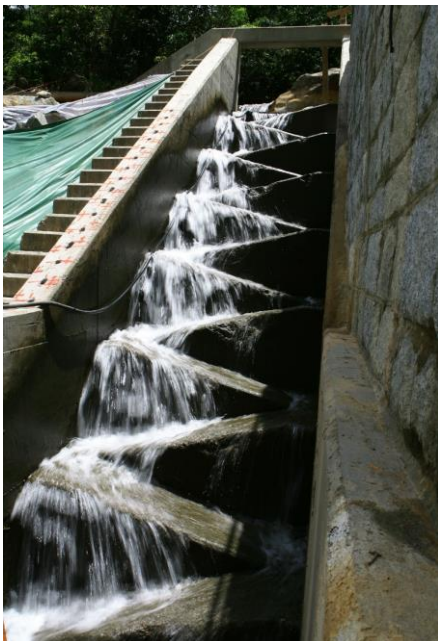
Figure 3.4: Zigzag ramps are constructed to lessen the environmental impacts of river training works
