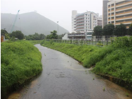
Figure 8.1: This channelised section will be revitalised into a River Park
