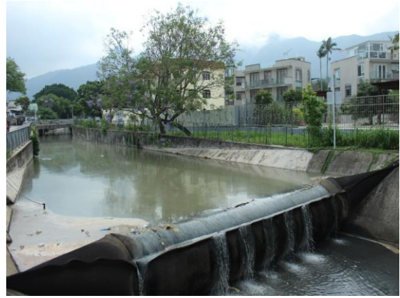
Figure 6.2: Inflatable fabridam at Wing Hing Wai
