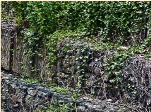
(2) Reinforcing grass lining in gabions
