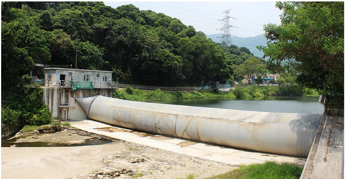
Inflatable fabric dam at Mui Shue Hang
