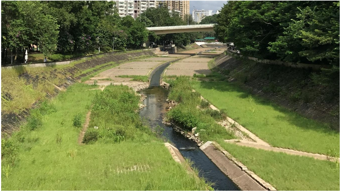
Eco-friendly river channel design at Tai Po Tau Shui Wai
